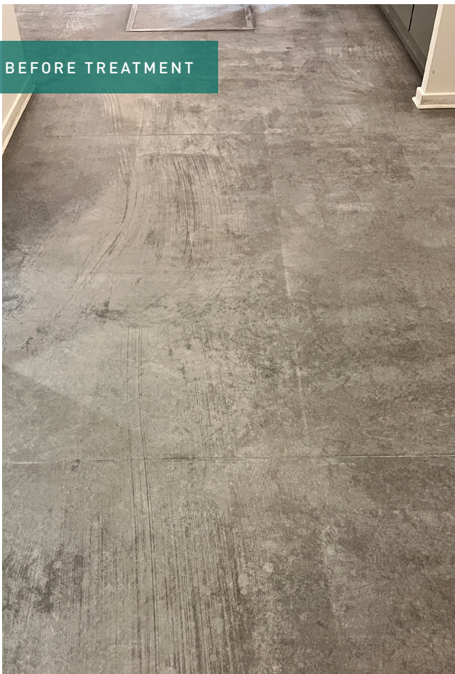
Corridor areas at a municipal heating plant - Treated with PUR Intensive Cleaner, sanded and finished with two coats of PUR Floor Sealer
